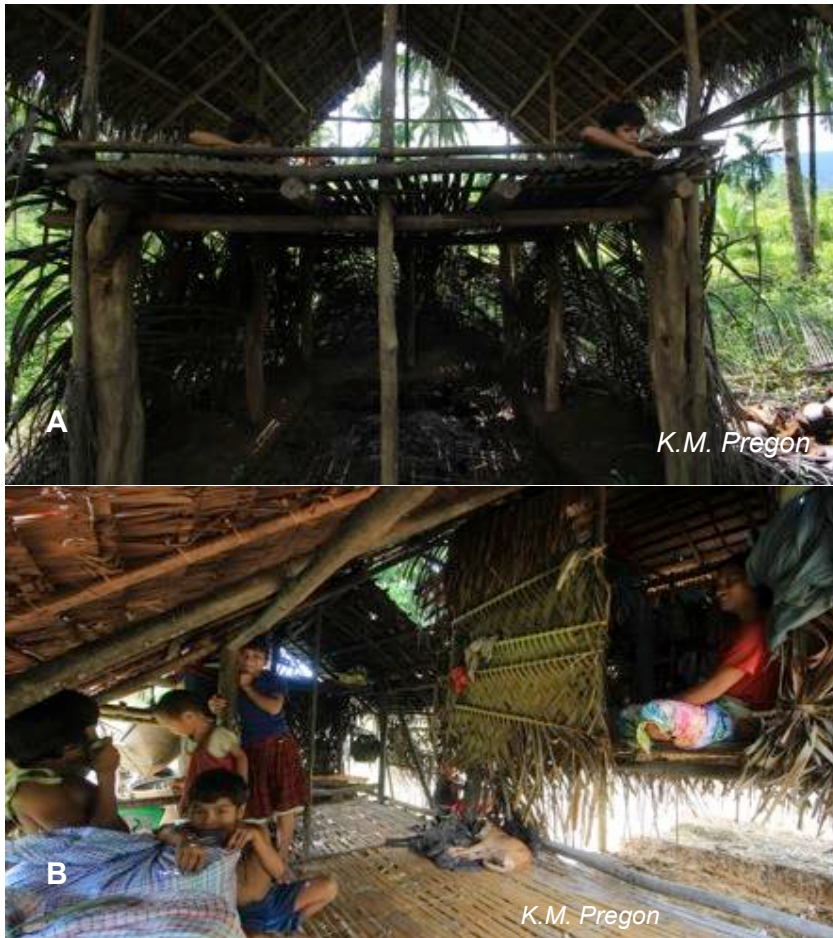
Plate 1. The community harvest timber products for house construction but they also use non-timber forest products such as Palm leaves and bamboo as building materials (Figure 6A and 6B.)
